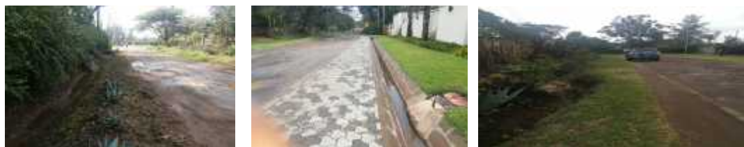
Photos of current status of the road
