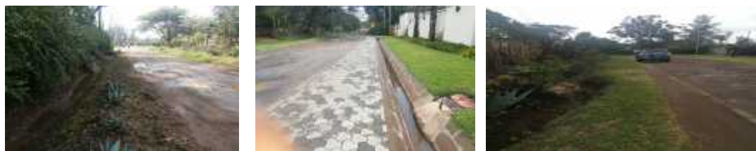
Photos of current status of the road
